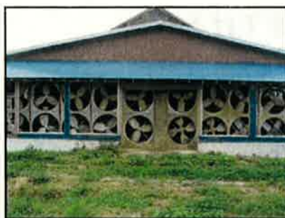
↑牛舎壁面の換気扇
